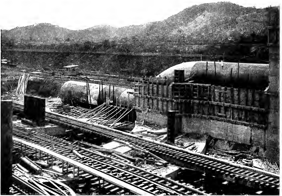
1. Section of the centre wall of Pedro Miguel Lock in course of construction, with culvert built into it. 2. Framework of the same culvert, showing how the water is passed down through a gigantic gooseneck from one level to another.
